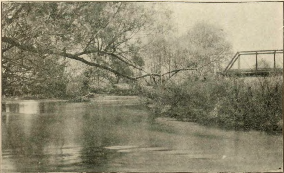
Alum Creek Bridge
