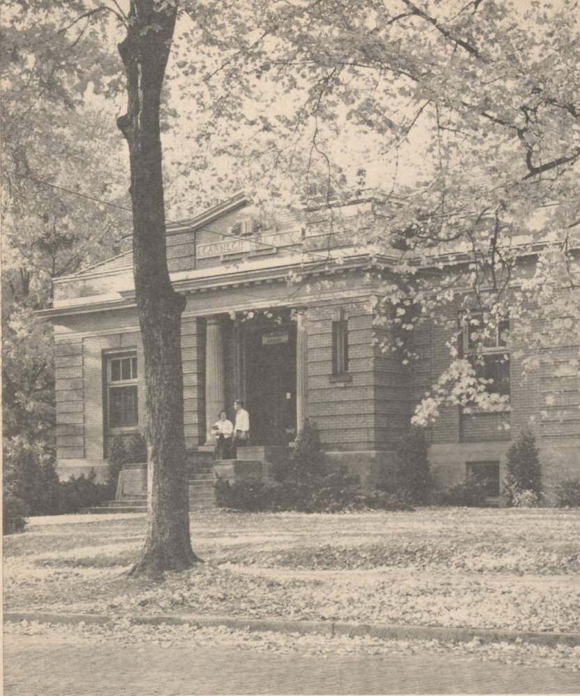
The Clippinger Administration Building
