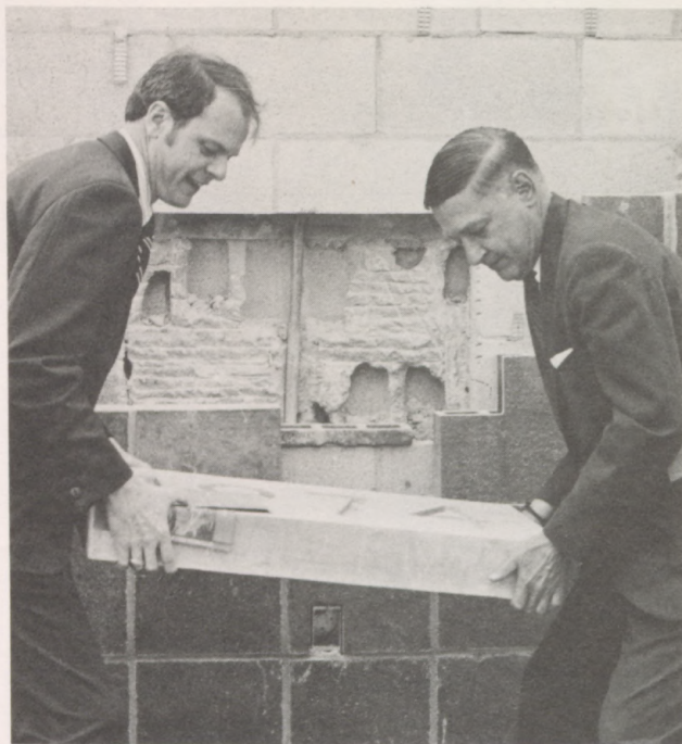
Among the bidding projects completed during Dr. Kerr's term of office was the Rike Physical Education and Recreation Center. Here, he and E.N. Funkhouser Jr., chairman of the Board of Trustees, place the building's cornerstone on June 1, 1974.
