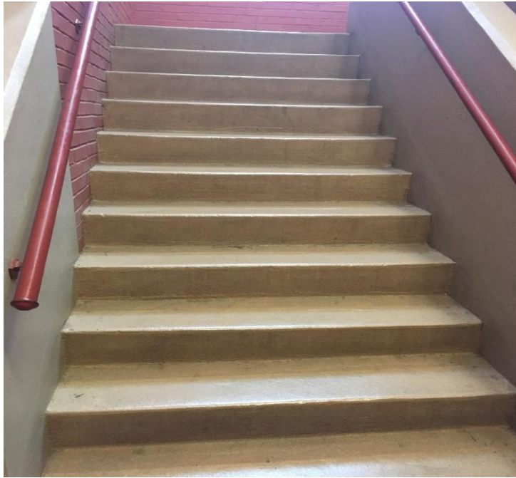
Figure A7: Towers Door 1 Inside
