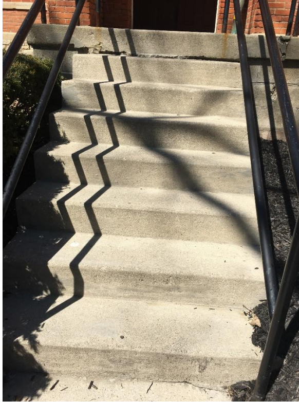
Figure A5: Towers Outside Door 2
