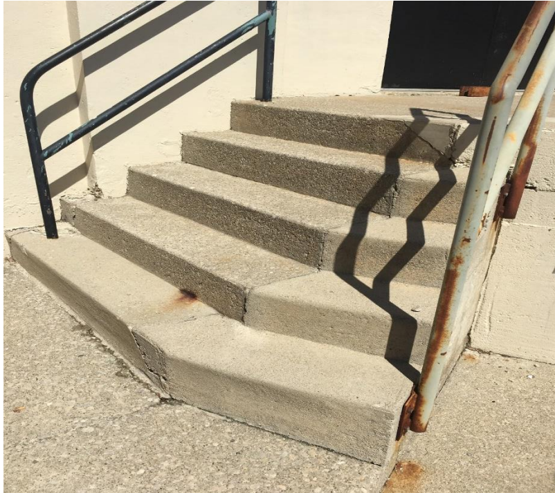
Figure A1: Music Building Outside Door 7
