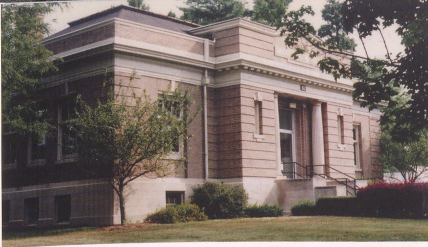
Otterbein's Carnegie Library now houses Admission offices. Opposite page: The Xenia Carnegie Library sat vacant for 25 years, but is now being renovated for private law offices.
