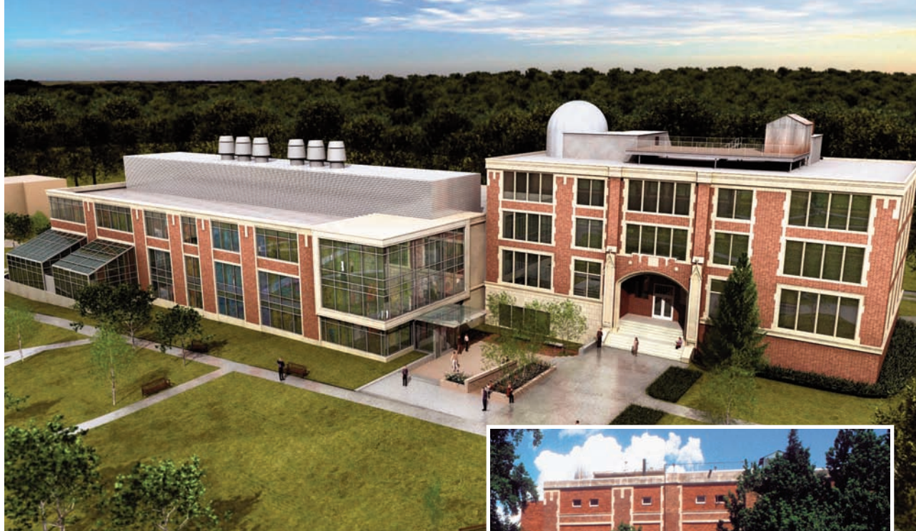
Above, a rendering of the planned new science complex, which will combine a renovation and expansion of the current Schear-McFadden Hall, which is shown in its current form at right.
